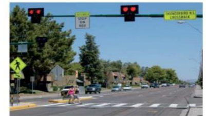
HAWK signal in Phoenix, AZ Source: Federal Highway Administration
